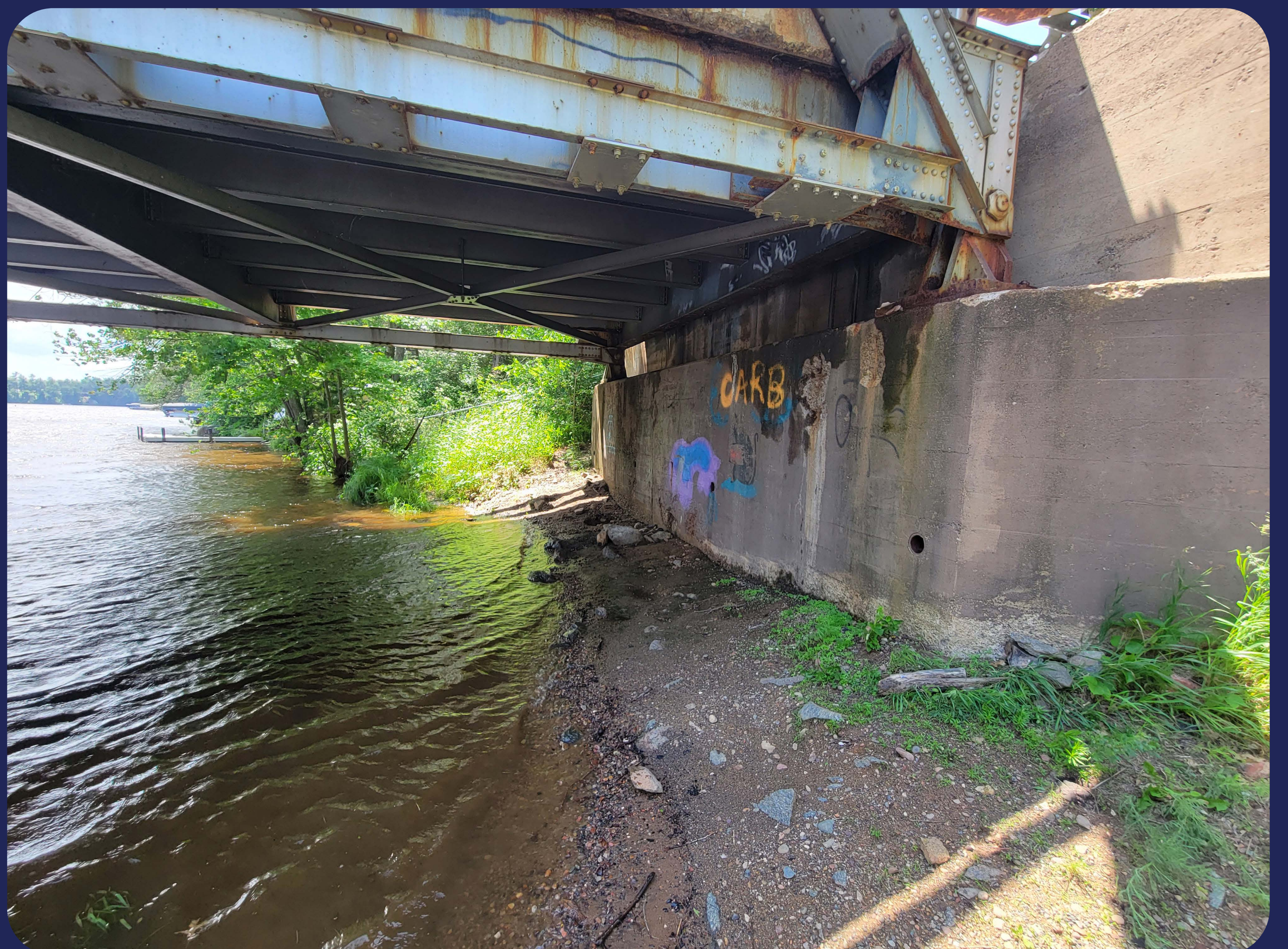
Concrete elements under the bridge exhibiting signs of deterioration
