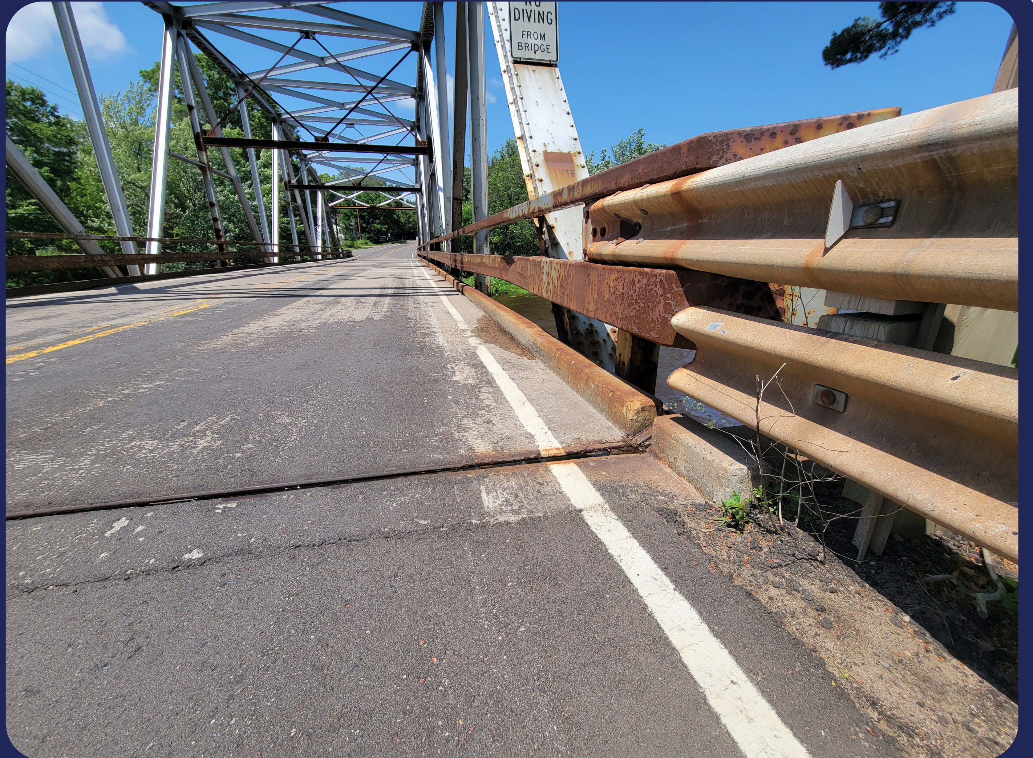
Steel elements showing corrosion
